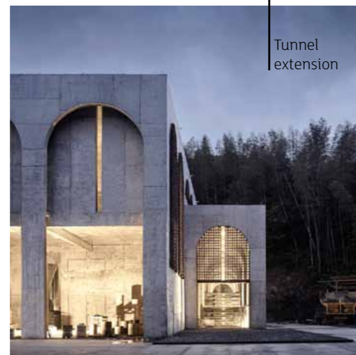
BingDing Wood Kiln Factory Renovation
